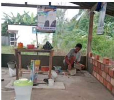
Gambar 11. Pekerjaan plester dinding pos kamling
