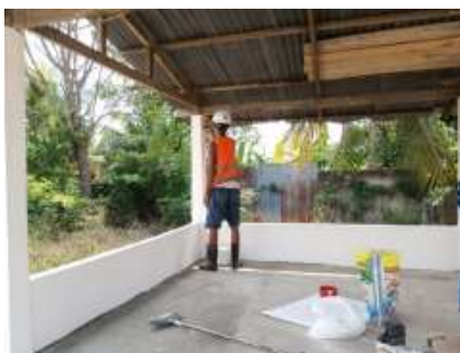
Gambar 12. Pekerjaan plester dinding pos kamling
