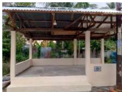
Gambar 12. Pekerjaan plester dinding pos kamling
